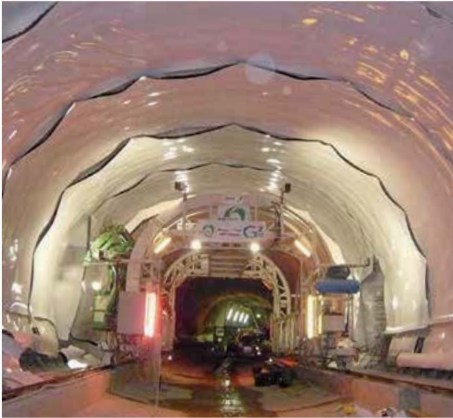
Tunnel PVC 2.5 mm
